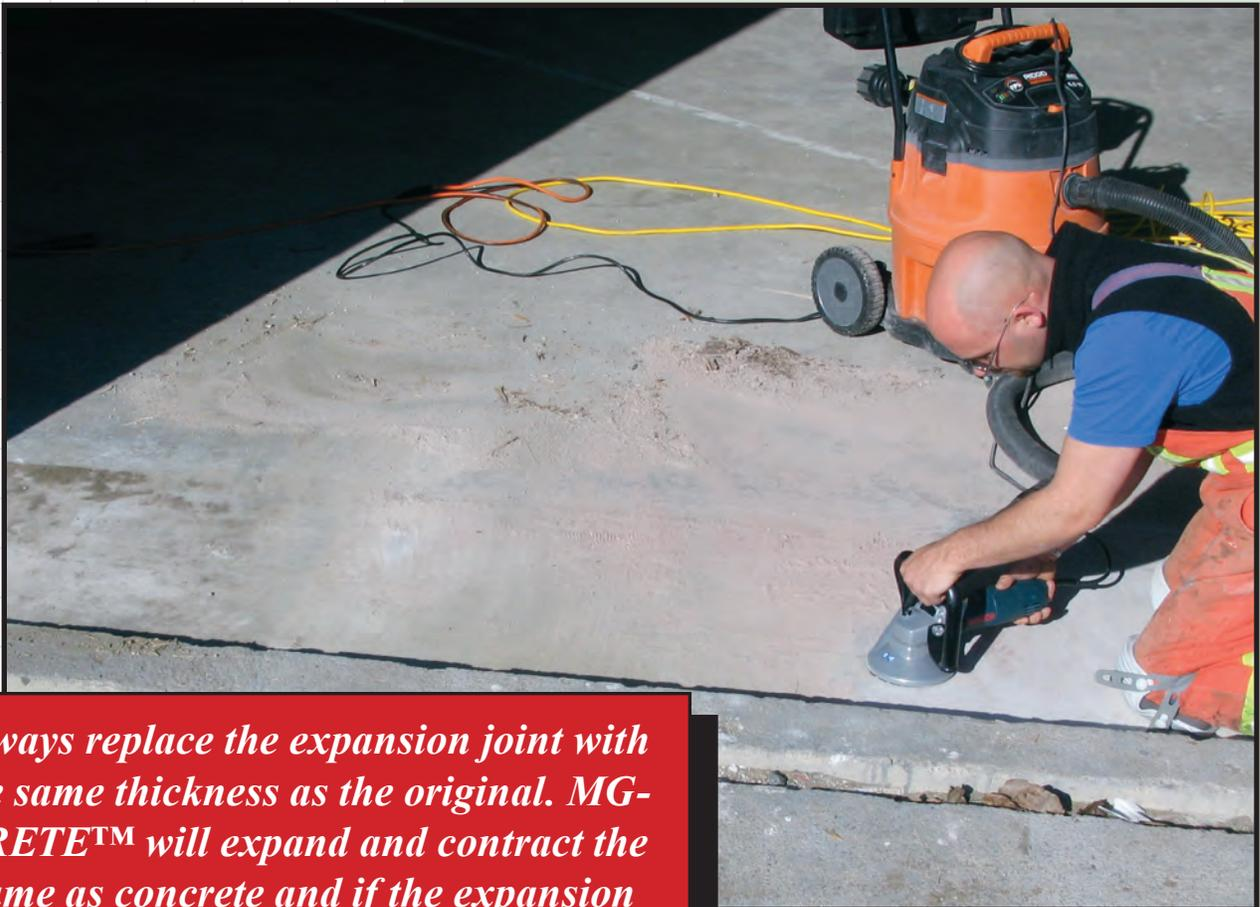
*Always replace the expansion joint with the same thickness as the original. MG-KRETE™ will expand and contract the same as concrete and if the expansion joint is not sufficient it will likely destroy the repair*
