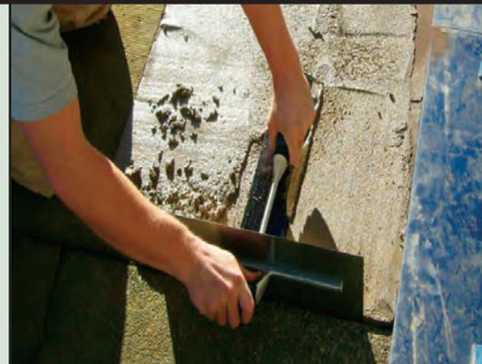
**When rebuilding edges be sure to make your mix dry enough so the MG-KRETE™ does not slump.**
