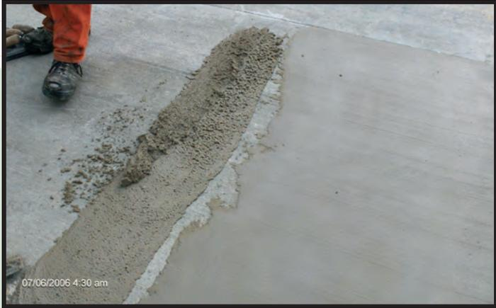
Many installers have great success with troweling half a bag at a time utilizing a second man for mixing only. When installing thin overlays it is important to consider substrate and air temperature and adjust set times accordingly so MG-KRETE™ can be troweled and finished before it begins to cure.
