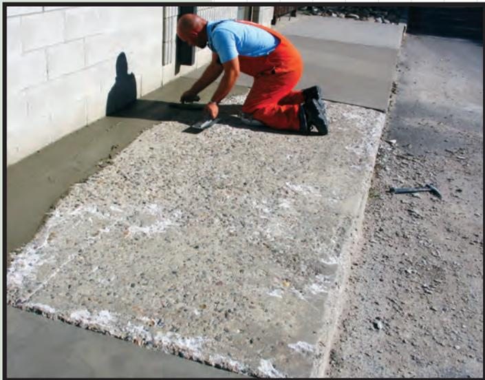
To avoid cold joints is easy if you are able to continually have new mixes ready once you have finished the last one. Simply spread the new mix along the area you just completed and trowel the new mix into the old.
